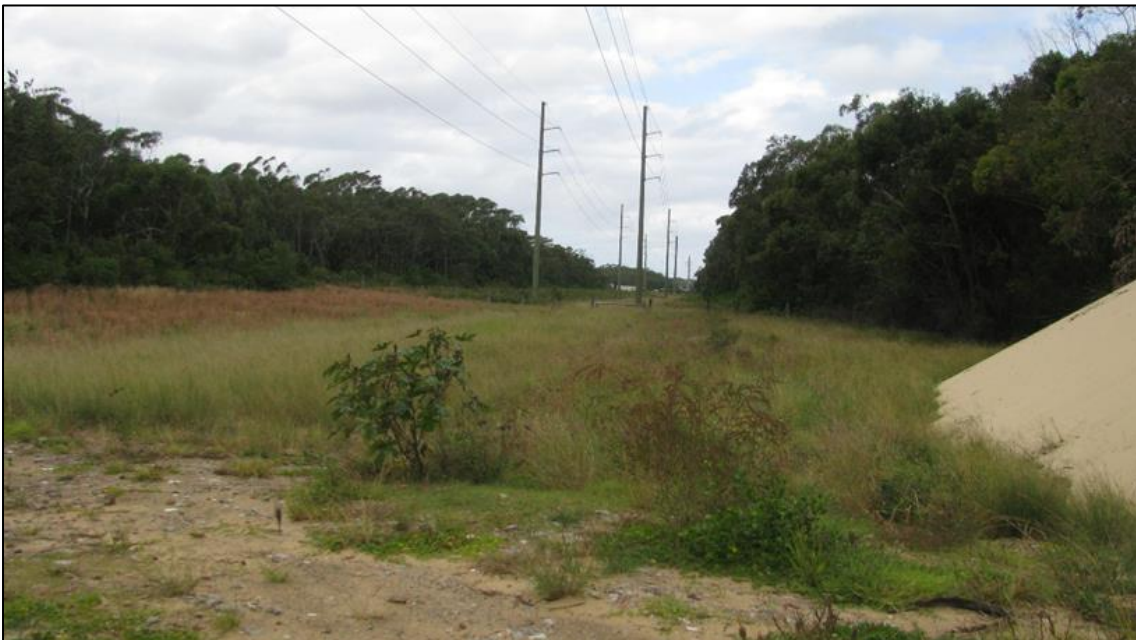
Photograph 4 – View East along 33kV Electricity Network: Poles, Wires, Easement and Part of Sand Incursion
