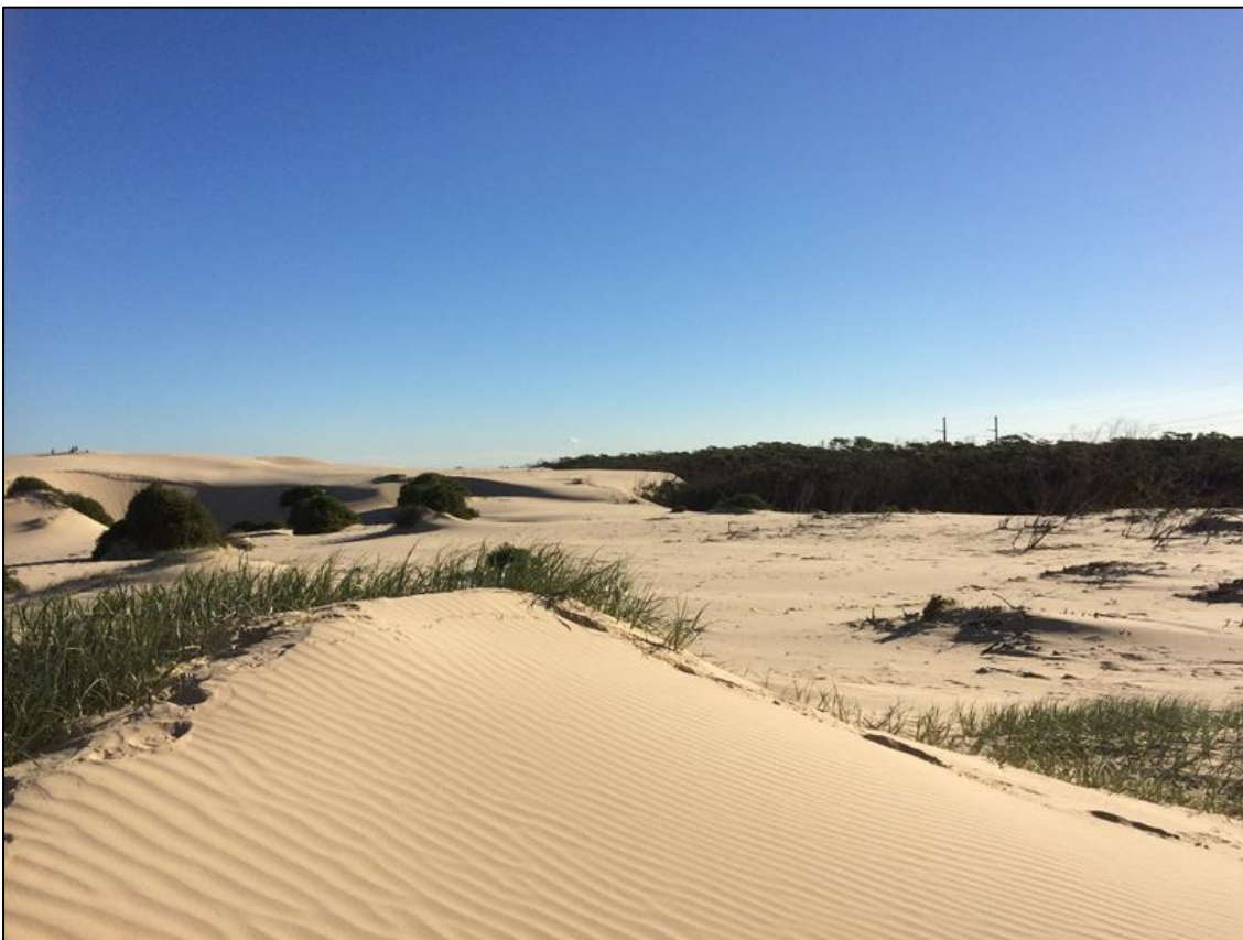
Photograph 2 – View North-West from Distant Sand Dunes: 33kV Electricity Network in Background
