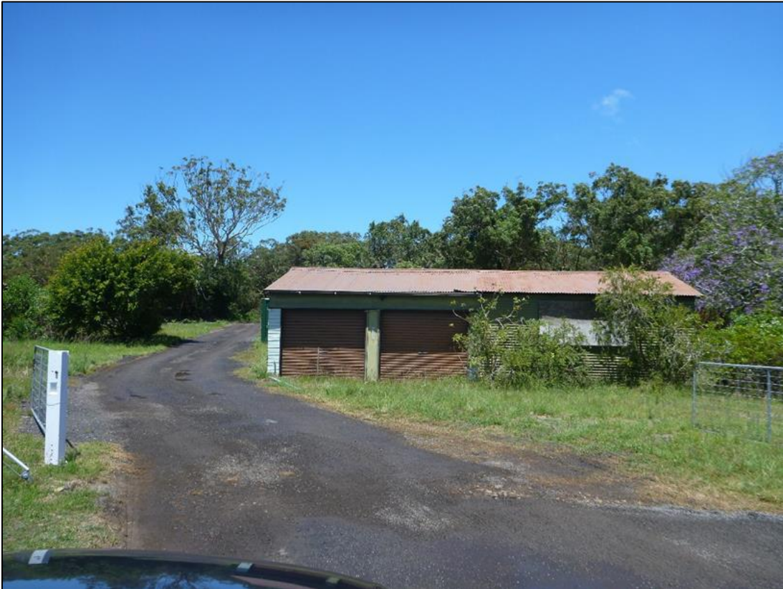
Photograph 1 – Site Access: View South into the Site at Intersection with Nelson Bay Road
